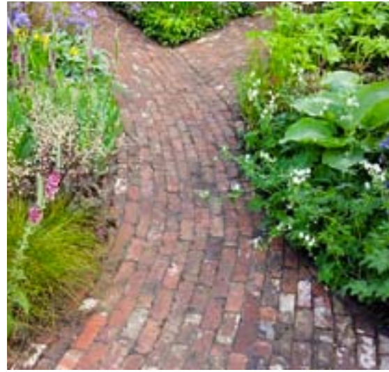
Brick pavers - running bond
