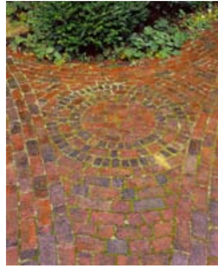
Brick pavers - patterning
