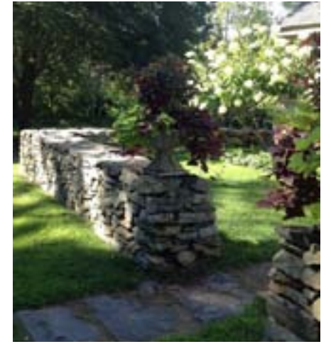
Stone wall - drystack
