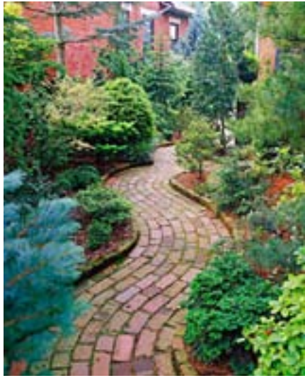
Brick pavers - running bond
