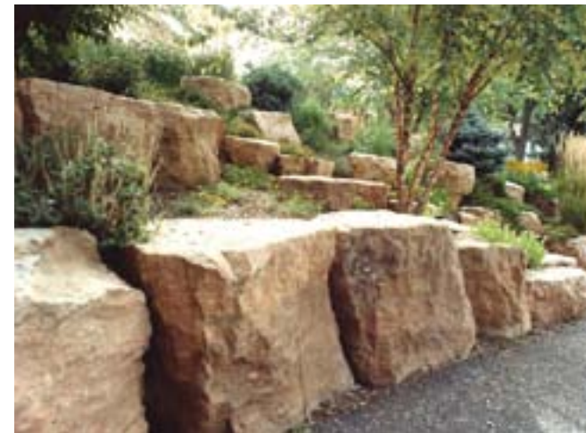
Stone outcropping - grade retention
