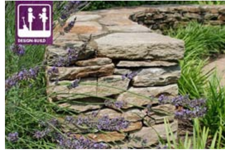
Stone wall - drystack, seat wall
