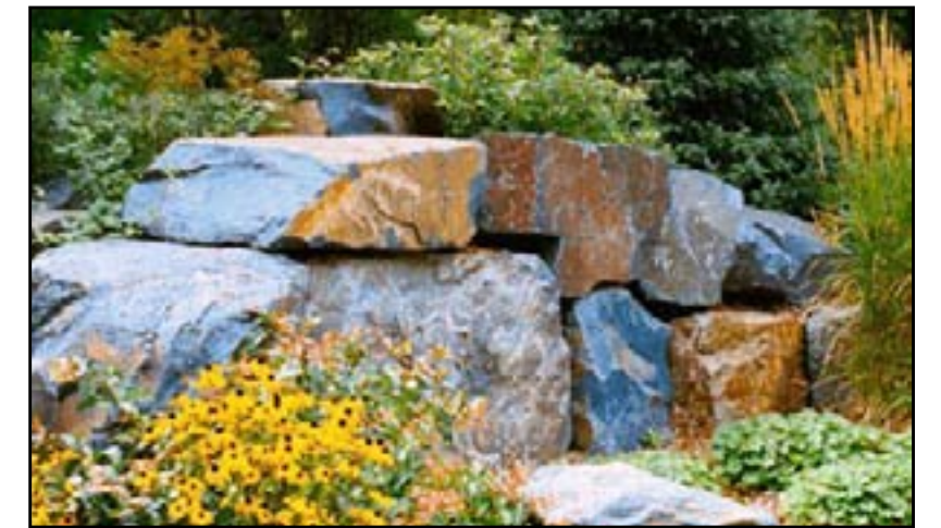
Stone outcropping - grade retention
